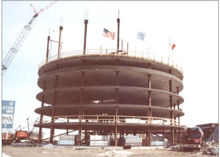
Figure 1 Lift slab construction of hotel tower in Portland, ME. Lifting is completed for the first tier of columns; second tier of columns with jacks on top are partially erected; slabs at top are temporarily parked.
