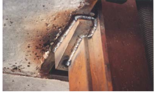
Figure 4 Wedges welded to weld block, column, and lifting collar.
