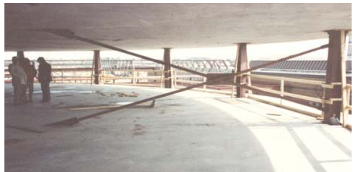
Figure 7 Typical radial braced frame.
