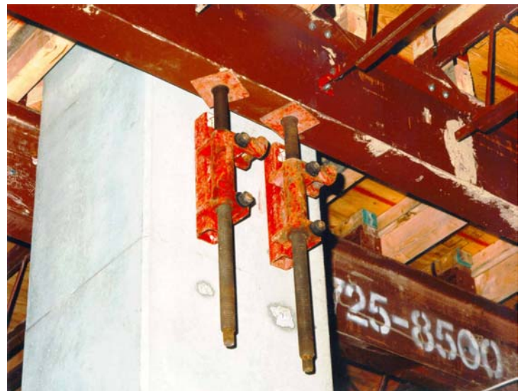
Figure 6. Support fixtures for flying forms.
